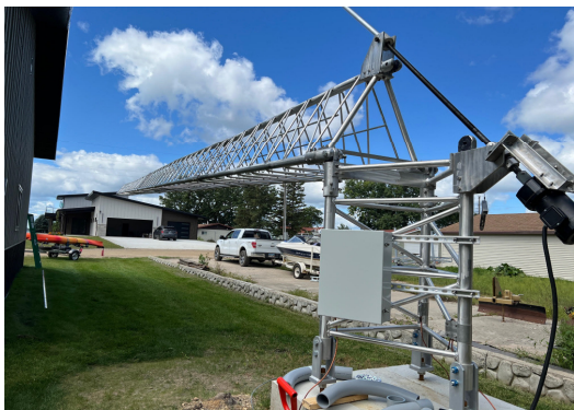
Heights Tower Ready to be “cranked” up
